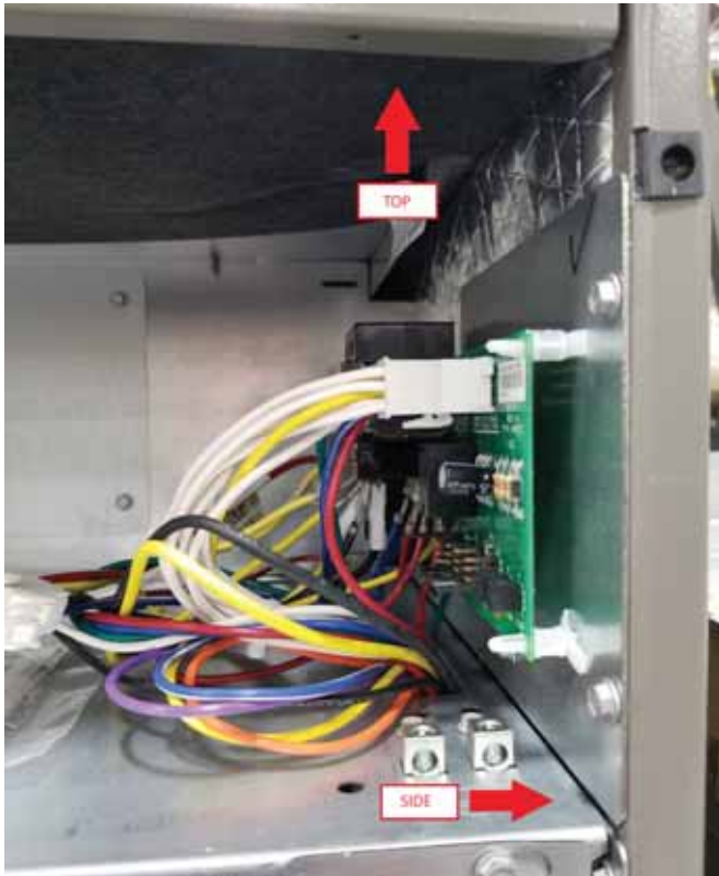
FIGURE 18. Electrical Connections (Upflow Configuration)
